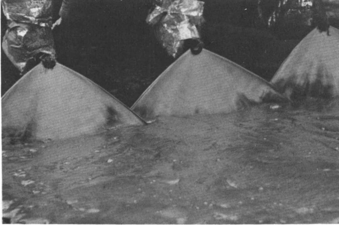
Figure 5. Sulfur foam being applied at 800 lb/min
