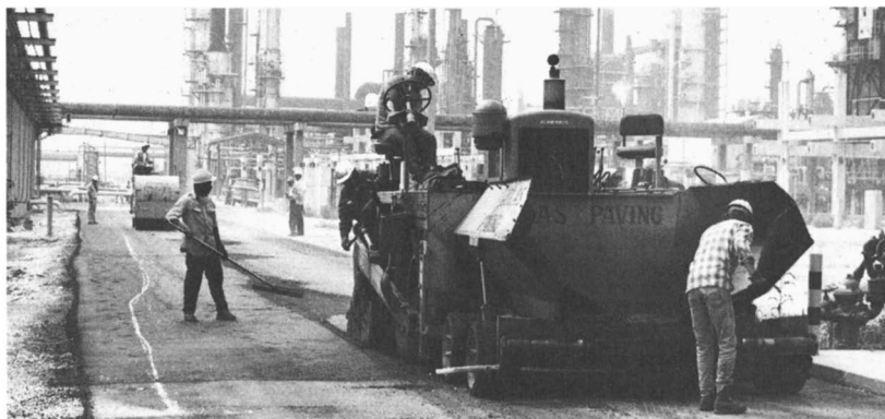
Figure 20. Placement and compaction of direct-substituted sulfur-asphalt paving in Ohio
