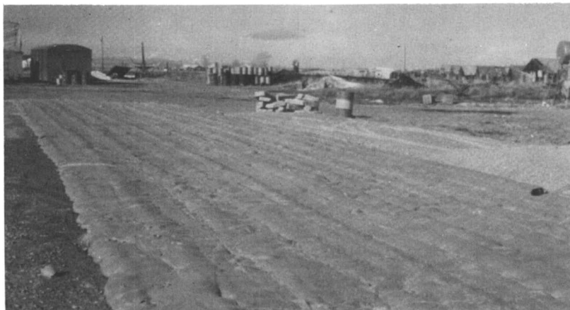
Figure 9. Two 10-ft wide and 150-ft long strips of 7-lb/ft 3 sulfur foam foamed in place side-by-side
