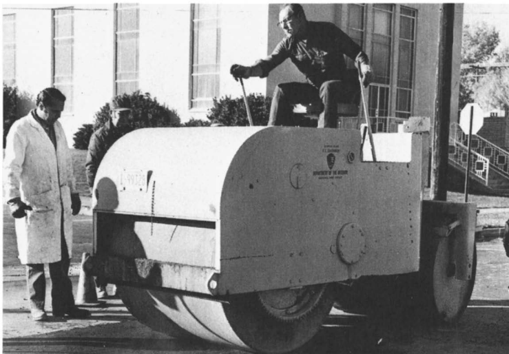
Figure 19. Laying patch of direct-substituted asphalt paving materials
